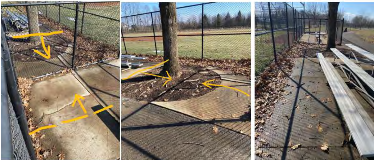
Third Base Dugout: Saw cut existing concrete, Grub out remaining stump and roots, install new concrete
