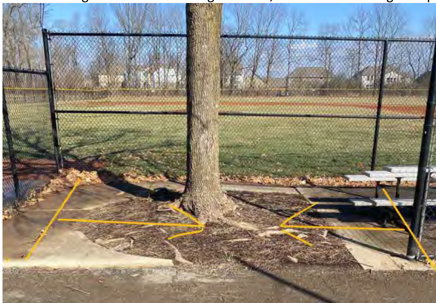
First Base Dugout: Saw cut existing concrete, Grub out remaining stump and roots, install new concrete.
